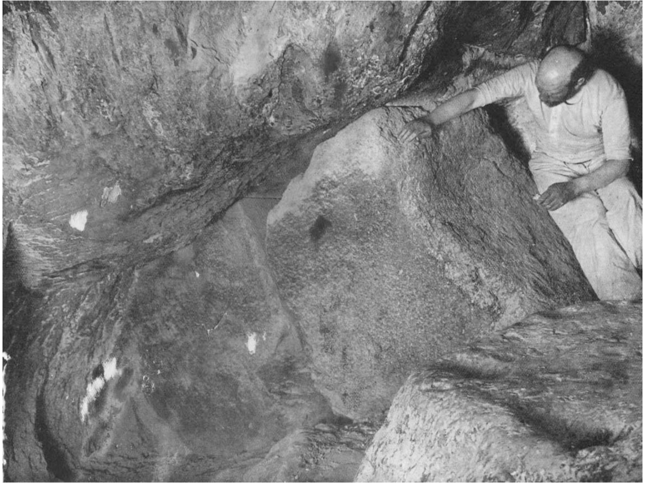
The upper south end, and portion of the west side of the GRANITE PLUG which completely blocks the lower end of the First Ascending Passage in the Great Pyramid of Gizeh; showing two of the series of three great stones, hidden in the Masonry for three thousands years, and exposed by Caliph Al Mamoun in the course of his excavations in the year 820 A.D.
