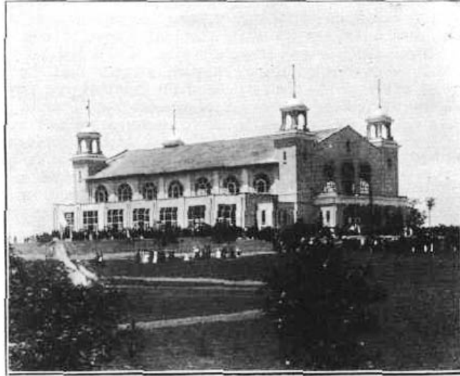
Exterior of Convention Hall, Hershey, Pa.
